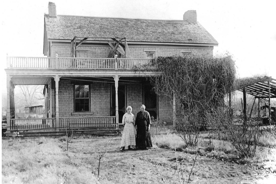
Brigham Whitmore house built @1882, Overton, NV. The house was built by early Mormon settlers using sun dried adobe brick. It featured a house plan with bisymmetry including two front entry doors, a style sometimes referred to as the architecture of polygamy.
